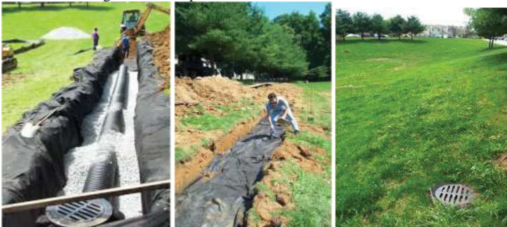
Figure 4: Example of Infiltration Trench Installation
