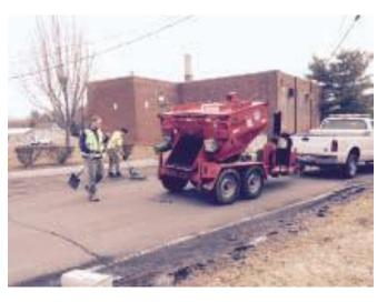
it hot for reuse in permanently filling and sealing potholes even on a cold day.
